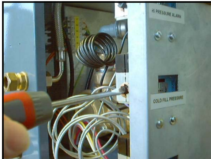
Figure 16. Pressure Switch Adjustment
